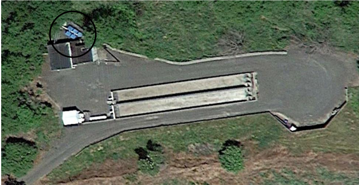
Figure 5-9. Existing Minthorn Springs Adult Lamprey Holding facility. Adults are held in tanks located in the black circle.
