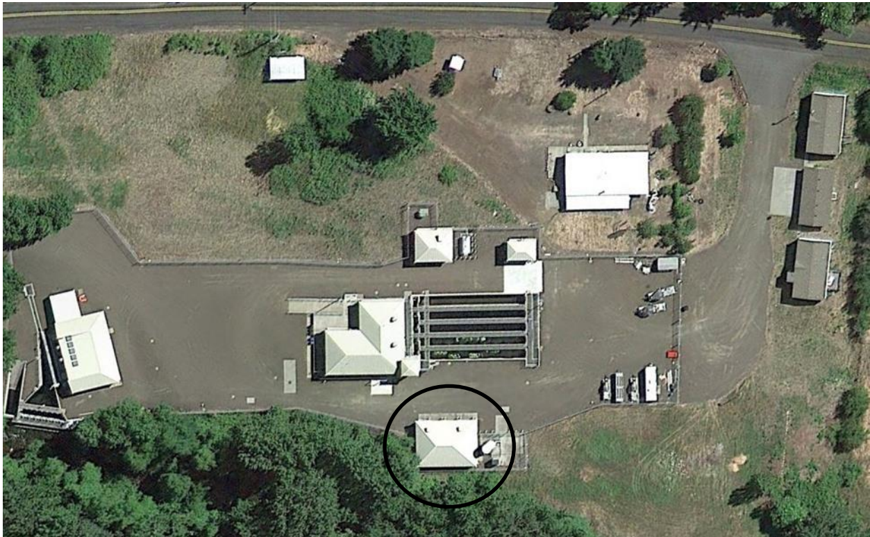
Figure 5-8. Existing South Fork Walla Walla Adult Holding Facility. The center-most pond is used for adult lamprey holding. Planned repurposed ozone building is in the black circle.
