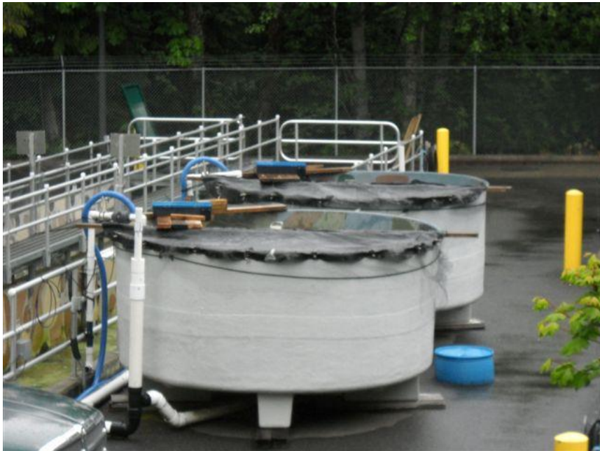
Figure 11: : Circular tanks at Parkdale Fish Facility used seasonally (late spring to early fall) for reconditioning kelts.
