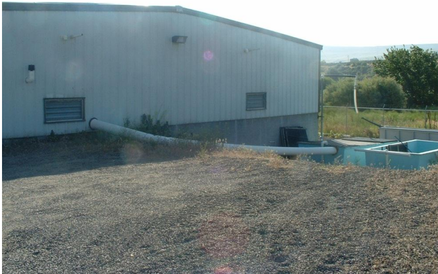
Figure 6. Chandler Juvenile Evaluation Facility PVC slide and holding tanks.
