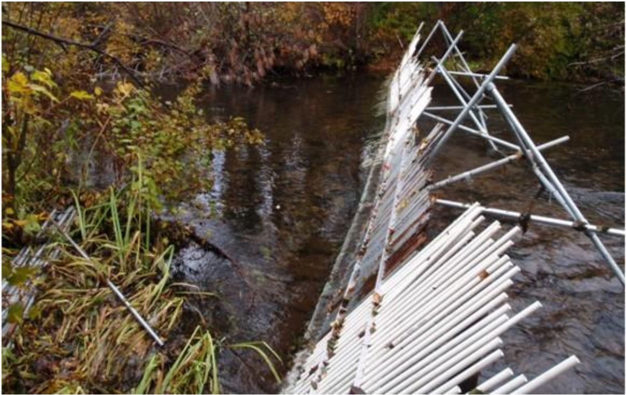
Figure 5. Mill Creek upstream weir RKM 30.2.
