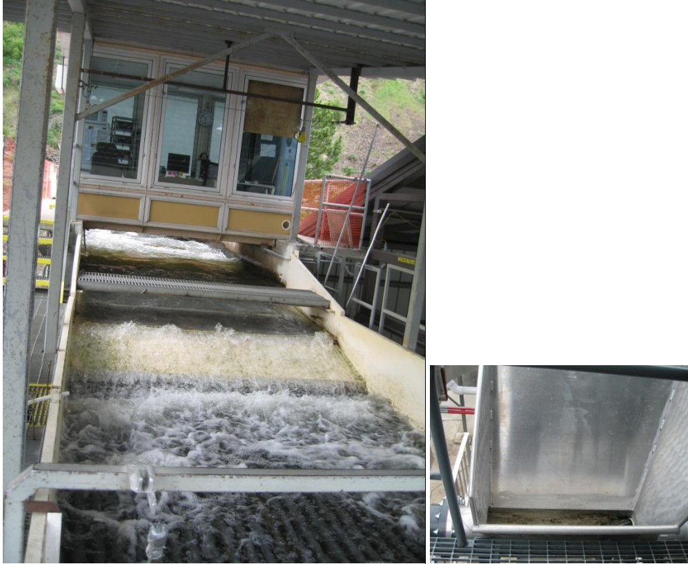
Figure 7: Juvenile bypass separator screen at Lower Granite Dam located on the lower Snake River. The photo on the right is the with kelt chute entrance where kelt are placed after being netted off of the separator screen.
