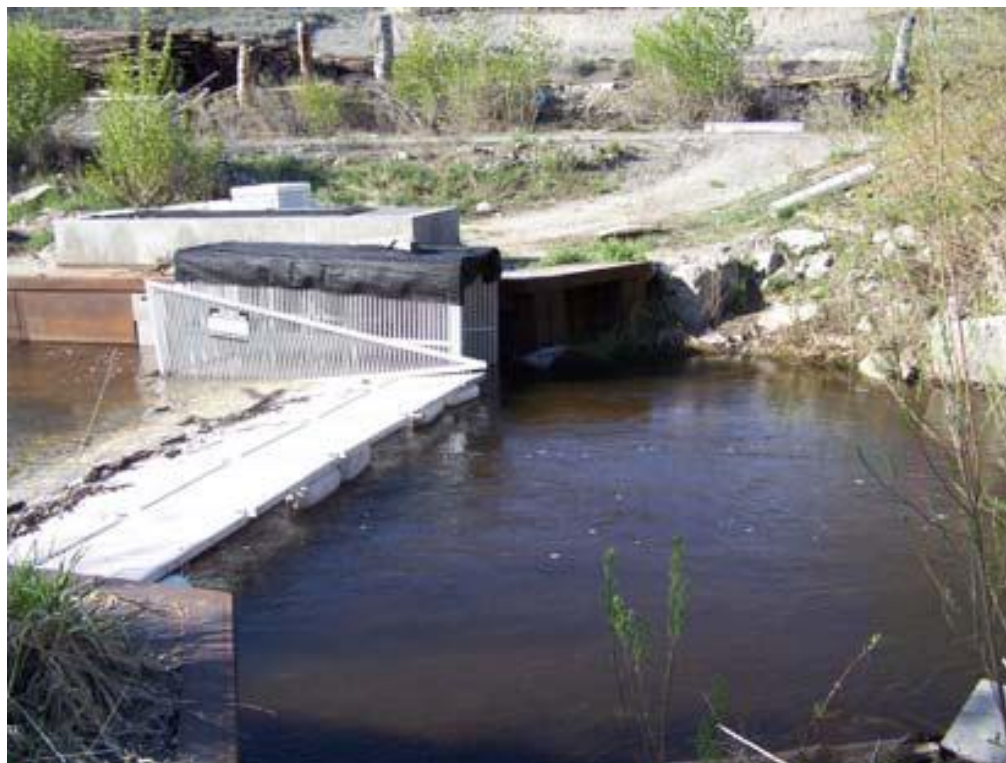
Figure 9: Resistance board weir located on Omak Creek.
