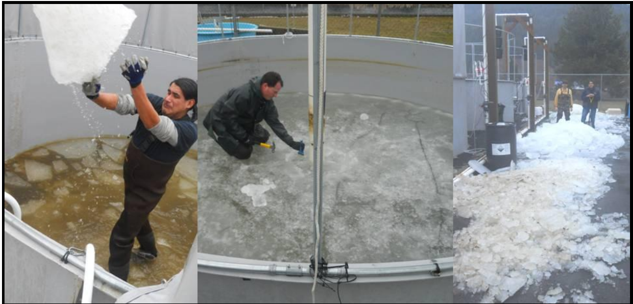
Figure 16. Ice was carefully removed by hand to avoid damaging the tanks. Several days of effort were necessary to clear the tanks and the out flow lines of all the ice.
