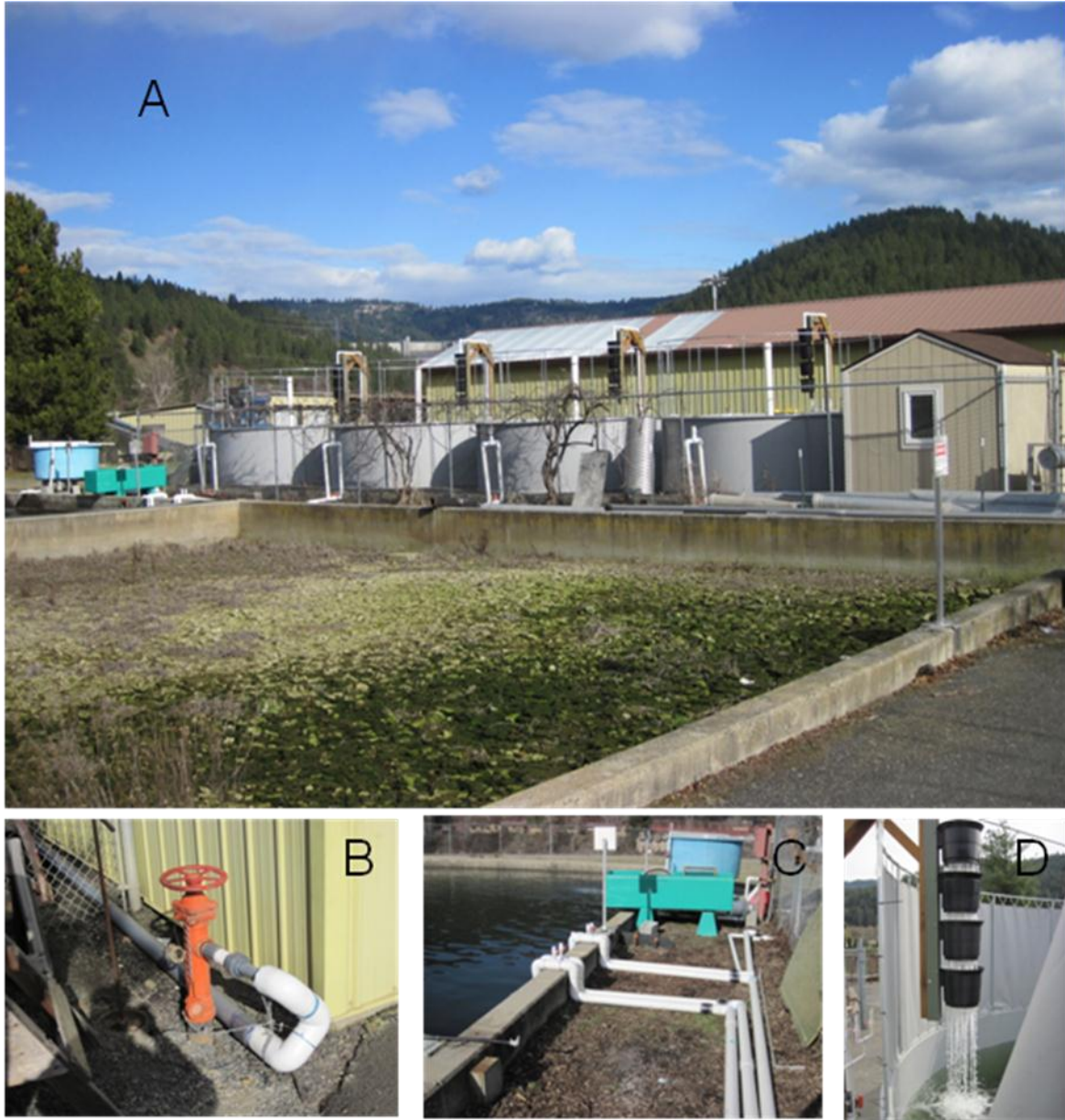
Figure 8: Experimental kelt conditioning tanks at Dworshak National Fish Hatchery. (A) Kelt tank overview. (B) Fire hydrant water supply. (C) Outflow to settling pond. (D) Four-bucket Koch ring degassing system in operation.
