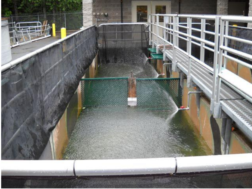
Figure 10: Parkdale Fish Facility raceways where kelts are held from late fall to early spring.
